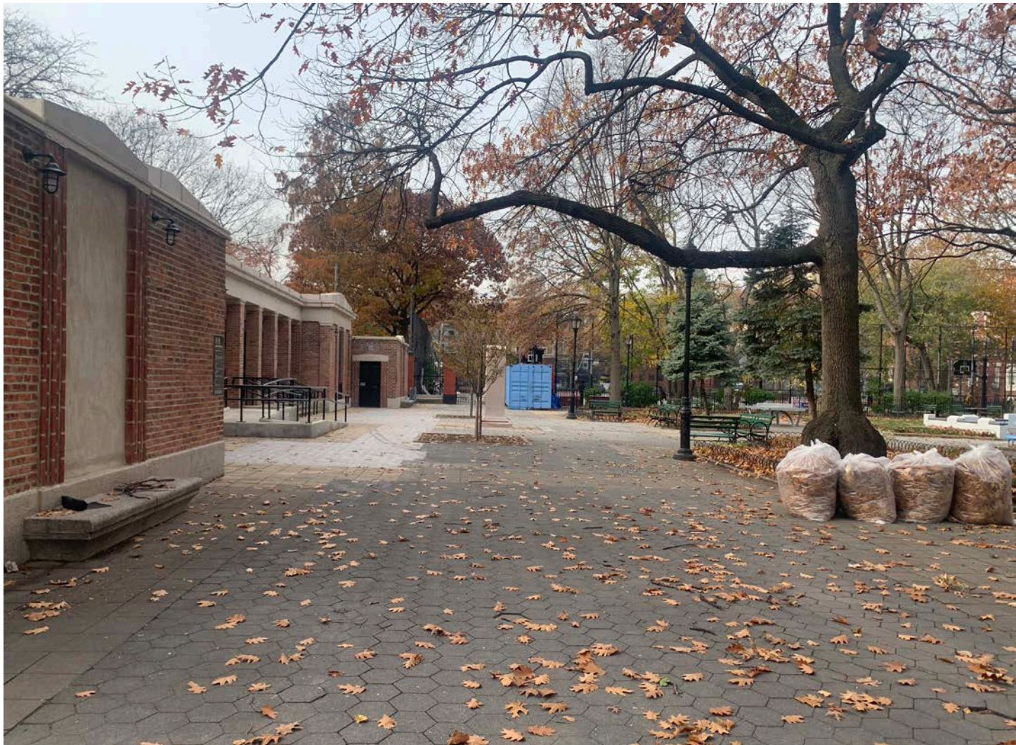
17 - Public Restrooms Boys & Girls Entrance Side
