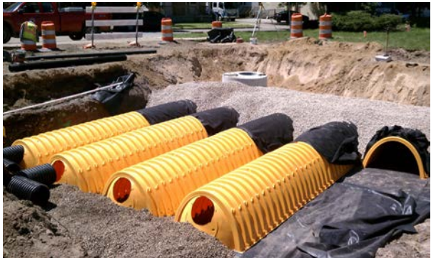
UNDERGROUND STORMWATER STORAGE SYSTEM
