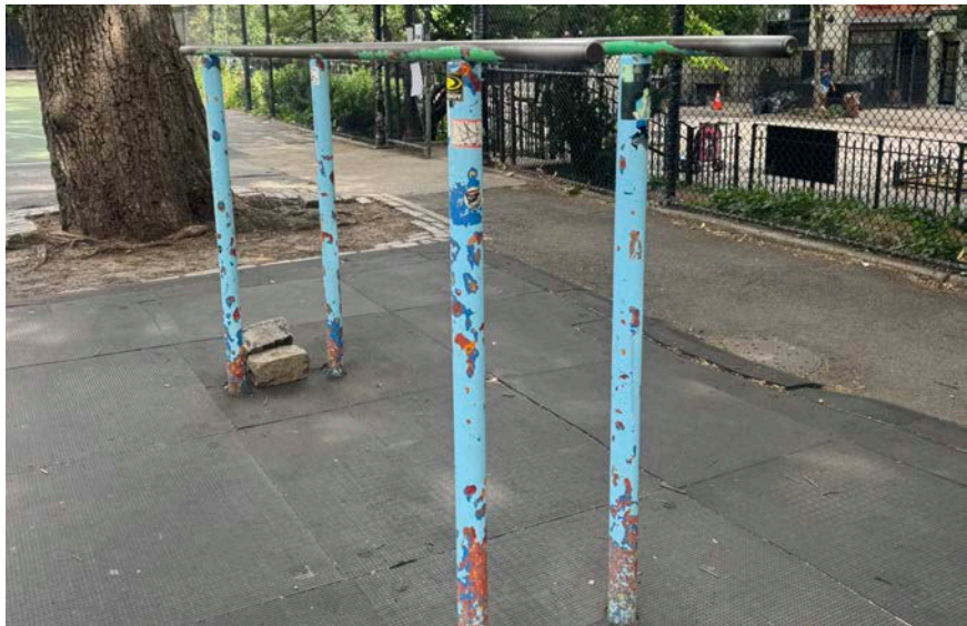
Fitness Blue Unit #1 Tall parallel bars with peeling paint & not ADA compliant
