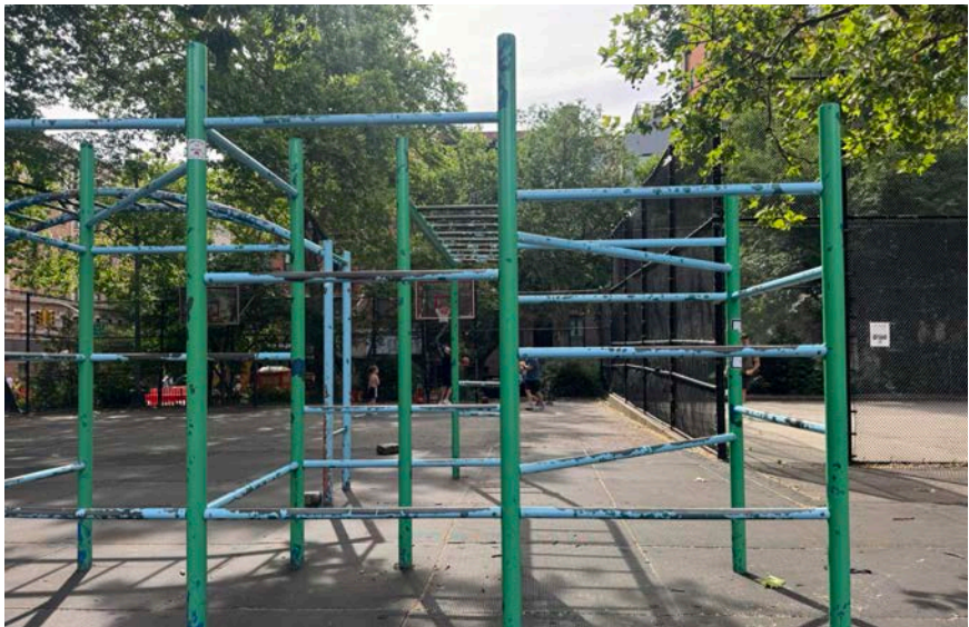
Fitness Green Unit #3 with peeling paint
